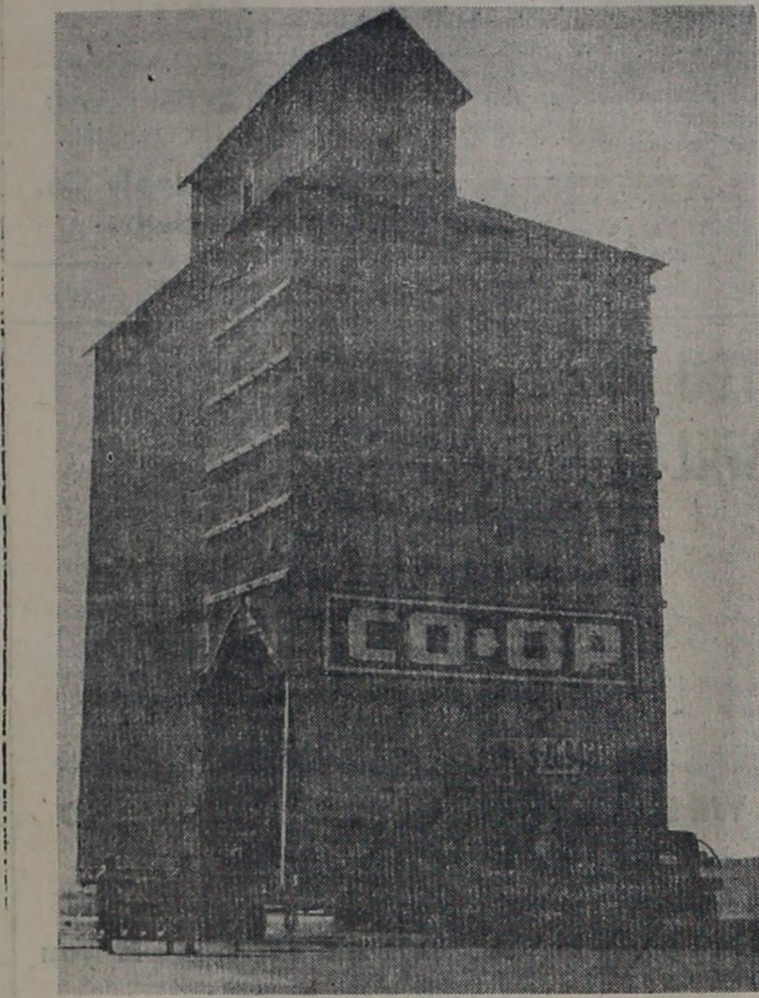
BIG MOVING JOB—Faith may remove mountains, but it remained for Homer Bennett, Clovis contractor, to demonstrate moving two large grain elevators from Clovis to Farwell, a distance of ten miles or more. Here we see one of the elevators, 76 feet in height, mounted on trucks and ready to "take off" across the country to its new location.
