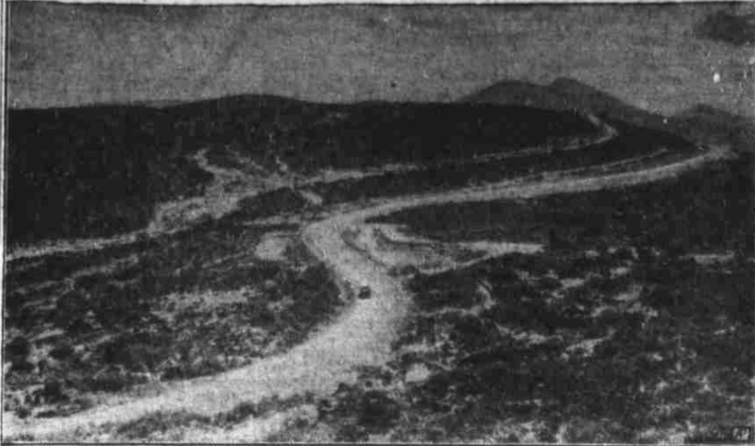
A trunk highway, running 700 miles from Laredo, Tex., to Mexico City, is to be formally opened by officials of the two
