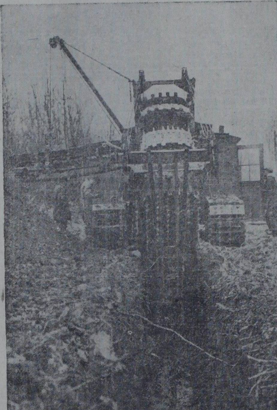
DIGGING THE "BIG DITCH" —A giant ditch-digger plows through Pennsylvania at a fast clip, taking everything in stride as it lays an oil pipe line to Northern cities from Texas oil fields.
