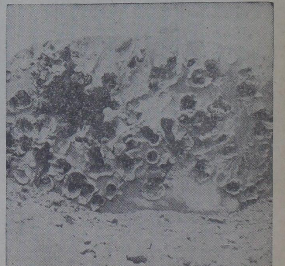
IMPREGNABLE —Allies preparing to invade France heard many stories about impregnable German fortifications. This perforated pillbox of concrete is mute testimony to German vulnerability. It also gives evidence of accuracy of American tank fire. (U. S. Army Photo).
