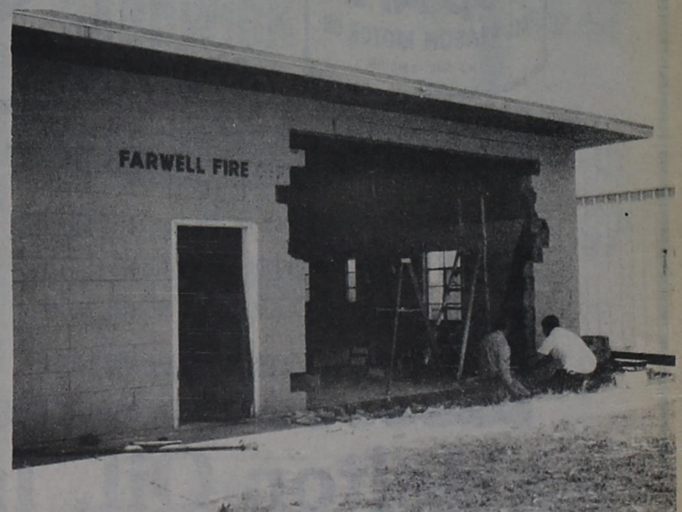
Building New Bay
