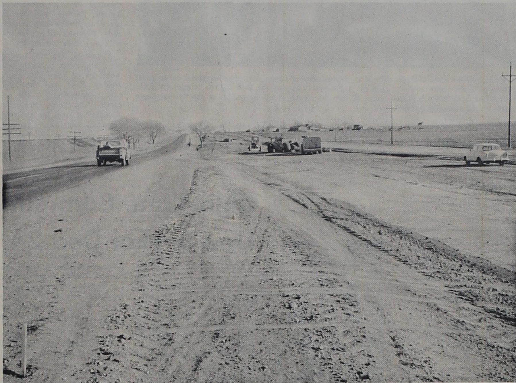
The old and the new lanes of U. S. Highways 70 and 84 will become one new highway southeast of Farwell and Texico when they are completed. Each lane will be 40 feet wide.
