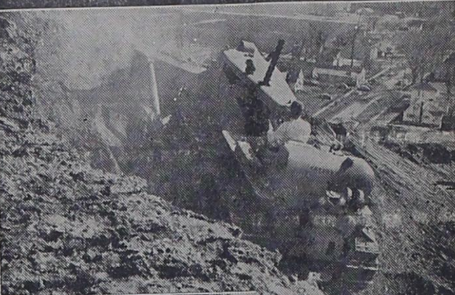
GOUGING Foothold on side of mine waste pile above Wenona, Ill., D8 prepares site for emergency warning radar station. (CNS PHOTO)
