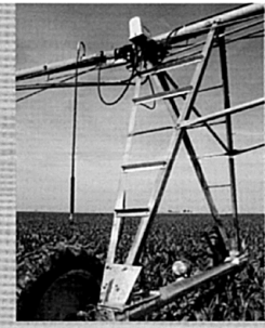
Valley Electric Conversion on a T-L
