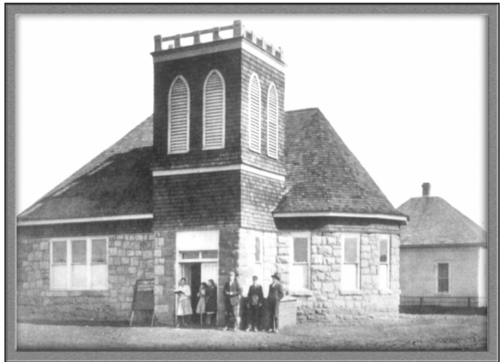
Congregational Church and parsonage at 1st Street and Avenue C. The rocks required to build it were hauled from Taiban, N.M.
