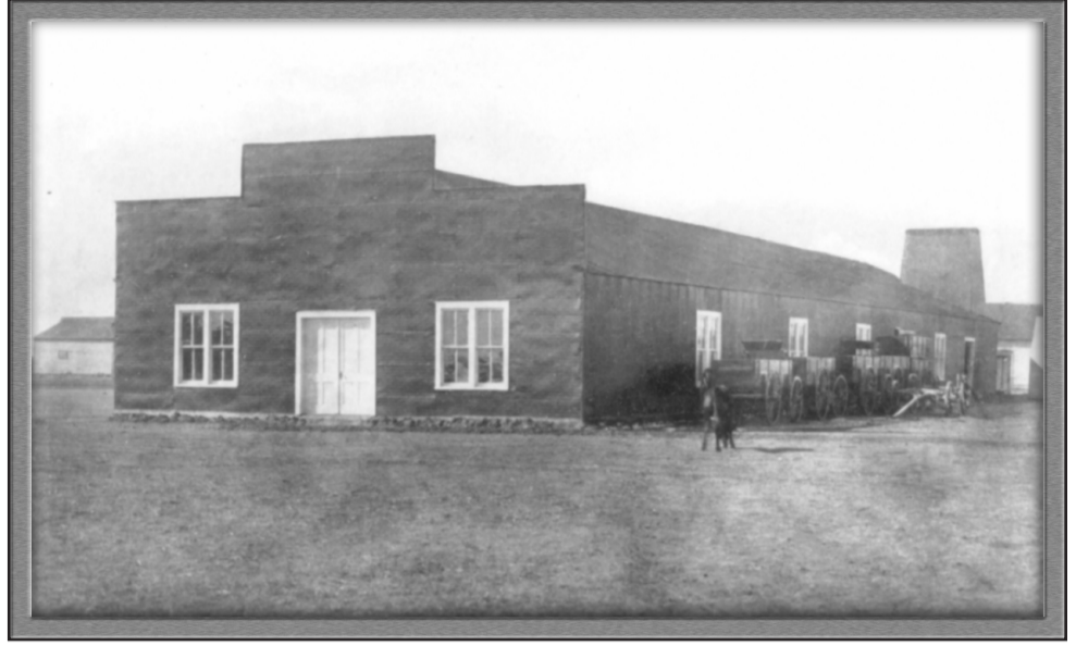
Corn shelling plant near the railroad tracks.
