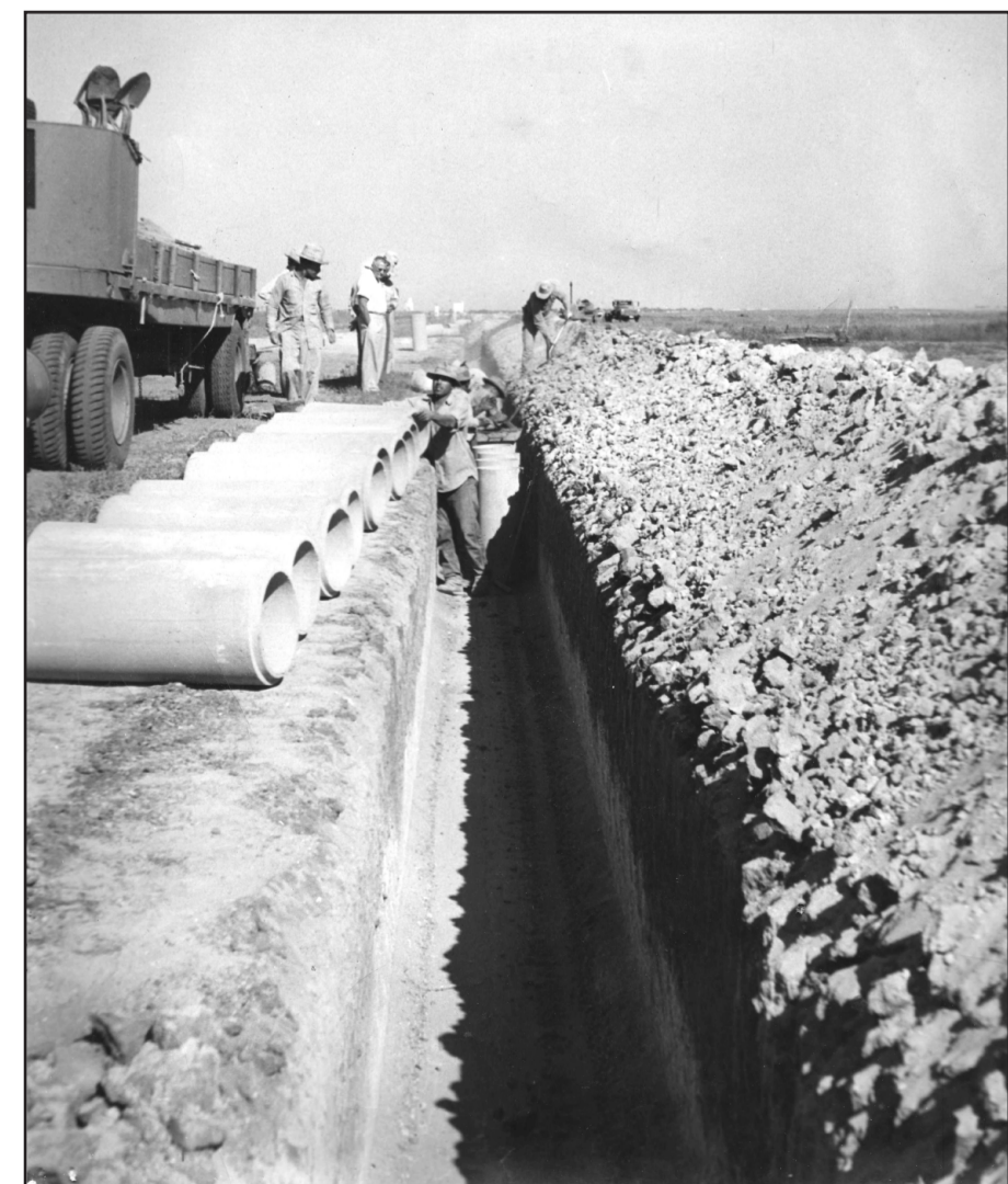
Miles of pipe were laid in the 1950's and 1960's.
