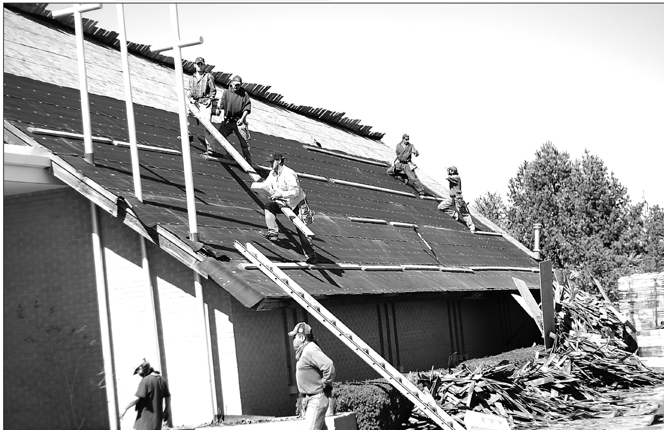
Hamlin Memorial United Methodist Church is getting a new roof.
