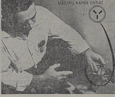
"All I'll have to do here is plug in my electric range. What's more, the wire used is #6 which means that the range will operate at top efficiency. Wire of the right size is an important part of electric appliance operation."
