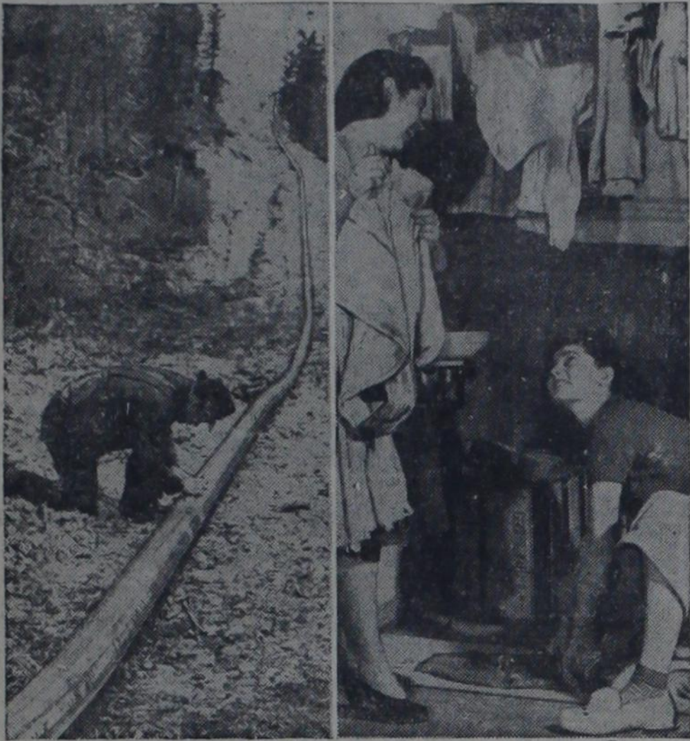
Oil for traffic using the new Alcan highway will be piped 550 miles from the huge underground lake of petroleum resources in the Mackenzie basin at Fort Norman. It will also serve ships along the Alaskan shore. Left: An inspector checks the welding on a section of the line. Right: Two of the many girls working in connection with the project are pictured in their laundry.
