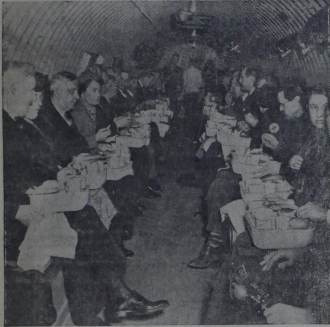
A luncheon served on air line trays publicly opened the bomb shelter by a large rubber concern at Akron, Ohio. This is a shatterproof flexible structure of the type tested by the war department. It is made of strong corrugated plates forming a gas and water-tight cylinder, and is large enough to accommodate 50 people.
