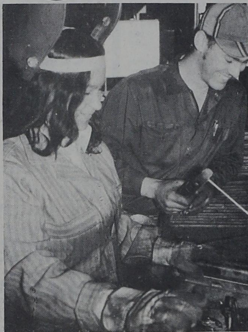
THIS IS THE WAY IT'S DONE - With her welding helmet pushed back on her head, Libby Cavallero watches Shop Foreman Tommy Crosswhite at Steel Products, Inc., as he prepares to show her the proper way to "tack" a plow part. The young Texico woman has recently been employed in the former all-male welding shop in Farwell.
