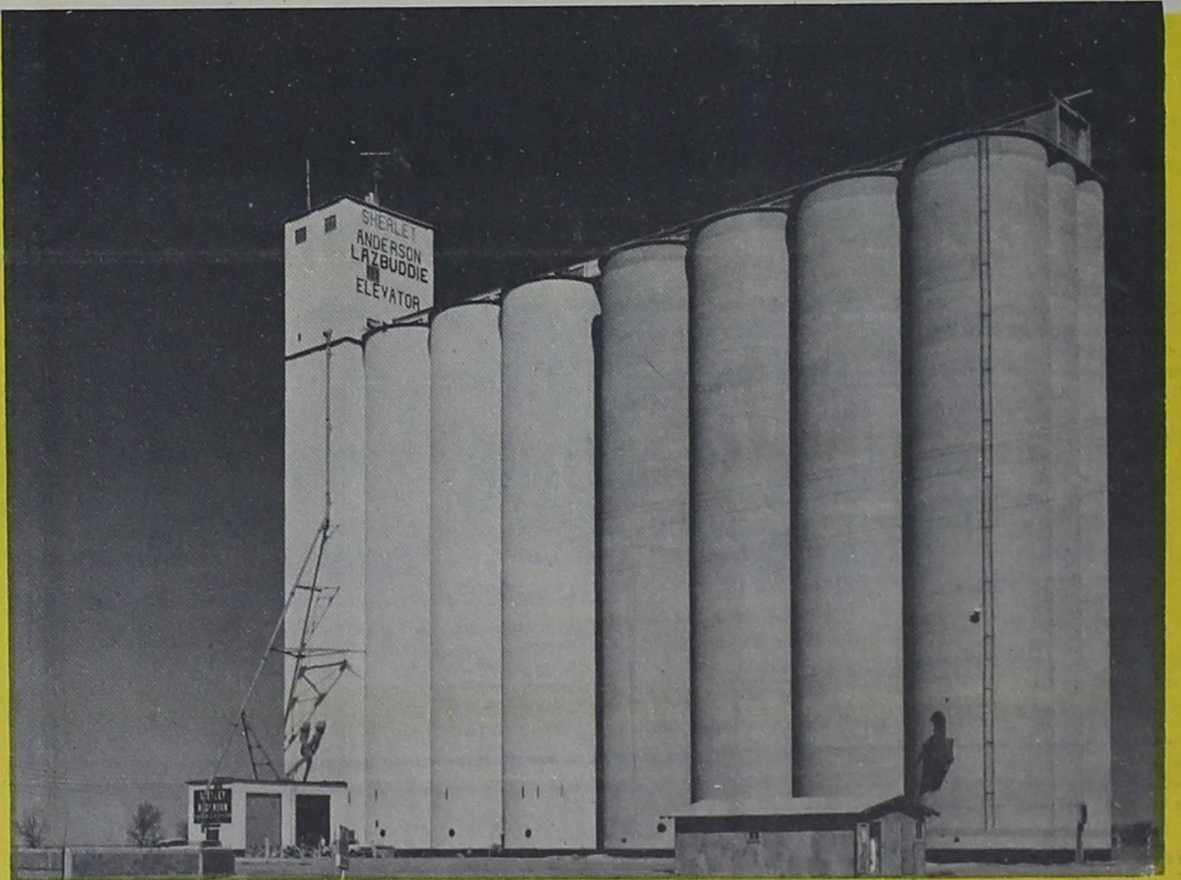
Sherley - Anderson LAZBUDDIE ELEVATOR
