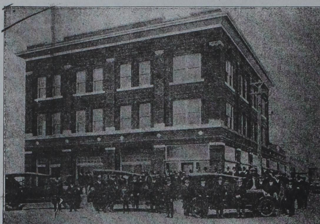
The Cannon Ball Motor Co. administration building in Texico.
