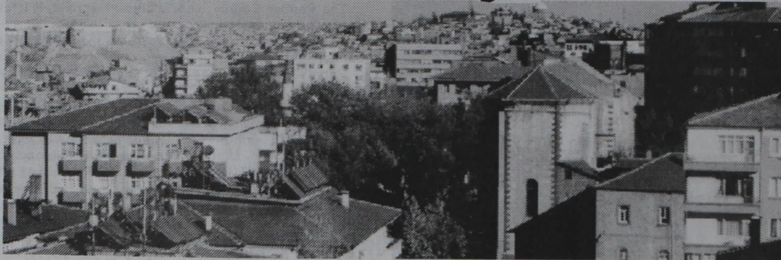
Almost every building in Istanbul is outfitted with solar powered water heaters. The advances in solar energy are being adapted more and more in structures throughout Turkey as a low cost and conservative energy source.
