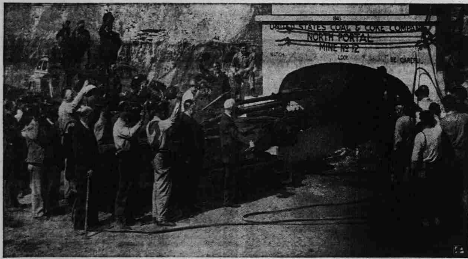
NEW COAL MINE 'IN THE SKY'—Atop a mountain near Gary, W. Va., workers stage a celebration as the cutting machine takes the first bite out of a seam of bituminous coal, visible in cliff at left.
