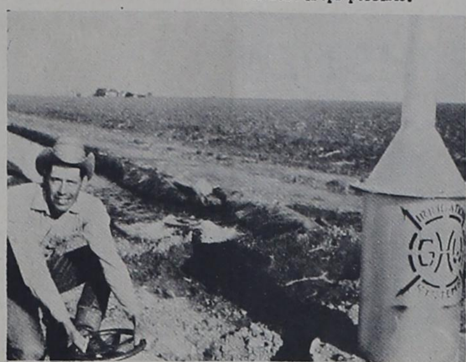
CONTROLLED FLOW OF WATER -- Weldon Crim turns the gate to separate or combine water from two or more wells in the same concrete pipeline.
