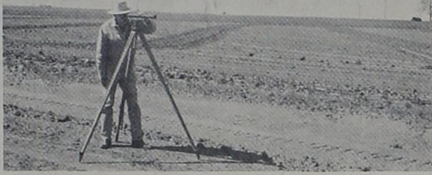
SCS technician Woodrow Fielder checks a waterway on the Joe Jones and John Aldridge farm at Lariat. This waterway was installed to safely dispose of excess run-off water. It will be sprigged to Midland Bermuda grass next month.
