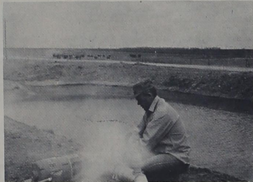
Jarrell Wright inspects his tail water return installation on the A. M. English farm west of Friona. This pit catches water from his farm and returns it through a plastic pipeline to the field for irrigation.
