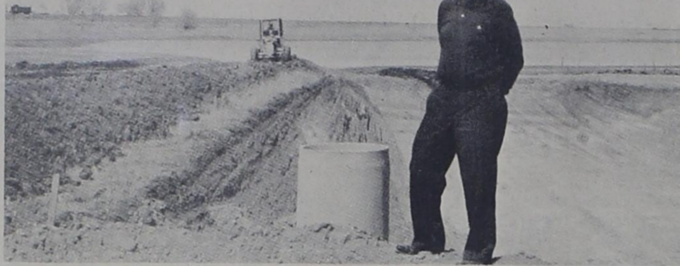
Sam Rundell of Farwell inspects tall water return installation on his farm southwest of Friona. This pit catches water from a playa lake and returns it through a high pressure plastic pipeline to the field for irrigation.
