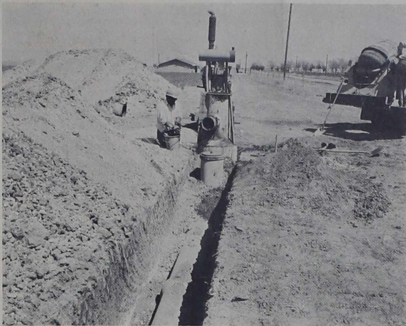
Irrigation pipeline being installed on Reagan Looney farm at Bovina. This line is being installed to conserve irrigation water and transport water from the well to the field.
