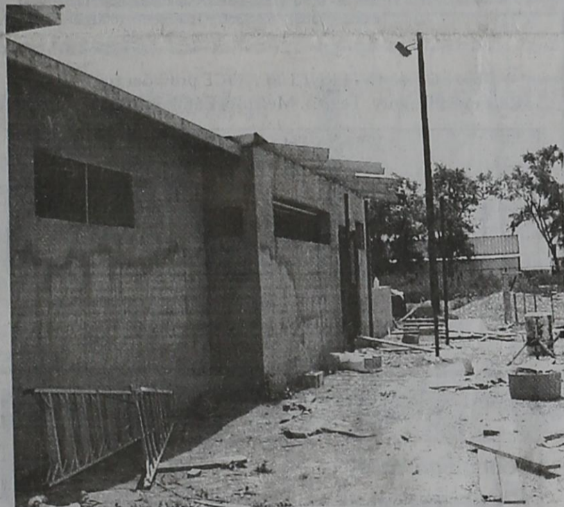
The cheese factory is still under construction.
