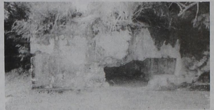
A destroyed Japanese pillbox on the beach.
