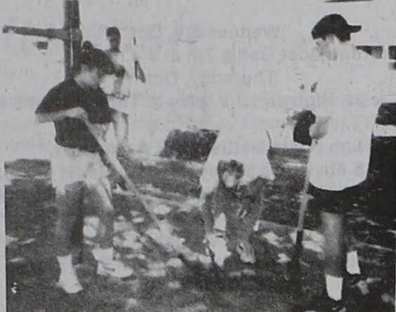
Lazbuddie High School National Honor Society members are shown working on the elementary school playground. The group worked Sept. 21 to move gravel into the new play area under newly-installed equipment. In back is Blake Mimms. In front are Shana Foster, Heath Brown and Brice Foster.
