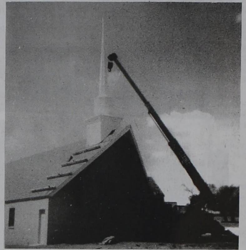
The new church steeple
