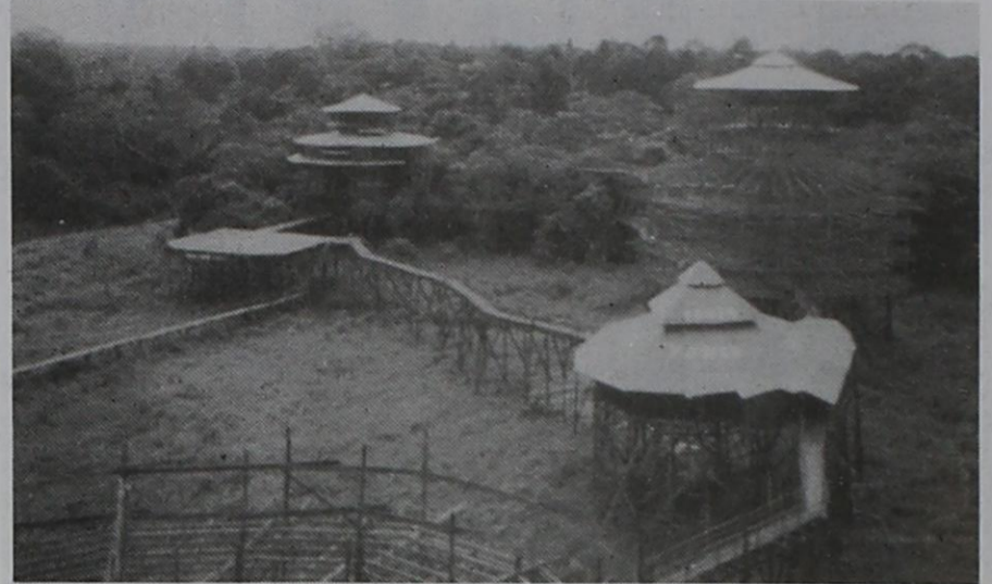
New construction on the fringe of the rainforest, which each new tower connected to the rest of the complex by bridges.
