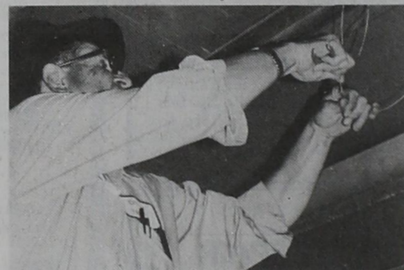
Dee Hammit sets up wiring at the gazebo.
