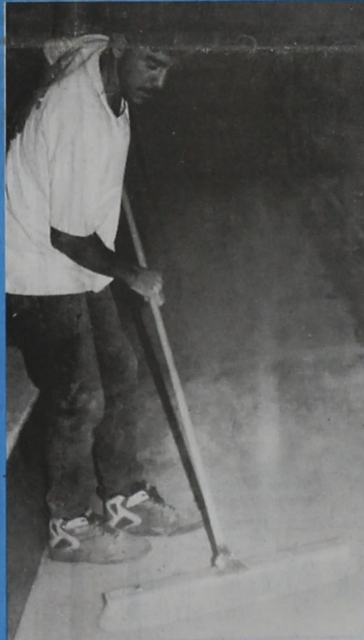
Joe Chavez sweeps the bleacher area of the new gym.
