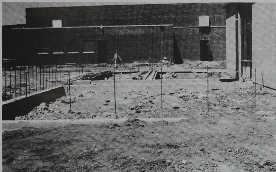
Construction continues on the Farwell school campus.
