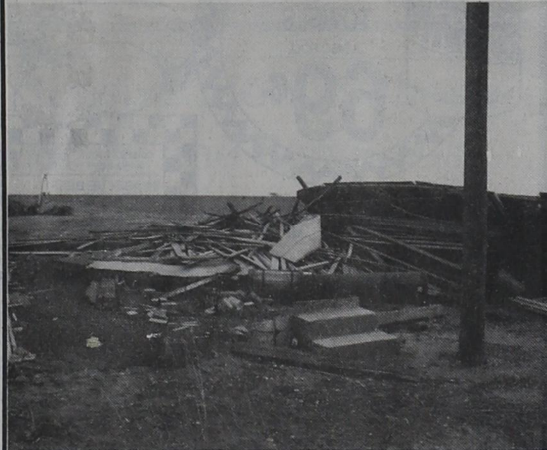
This storage barn on the old Hassell property was demolished.
