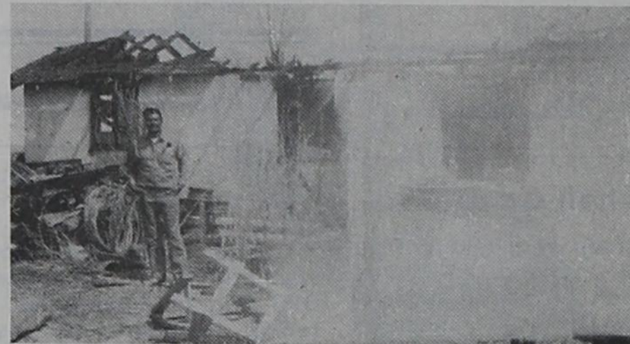
Lewis Foster stands beside the storage building on the north edge of Farwell that burned Monday night. It belonged to the New Light Baptist Church.
