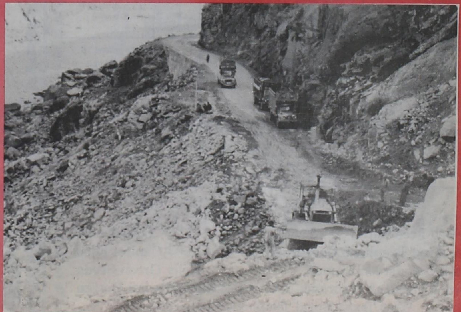
The Pakistani Army cut a path through the rockslide.
