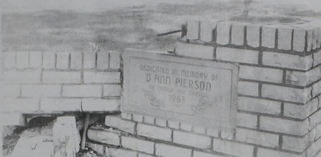
This brick water fountain dedicated to D'Ann Pierson was a casualty of the Farwell school construction program. Pierson, daughter of Mr. and Mrs. Steve Pierson of Oklahoma Lane, died in an accident in March 1983 while was a student at Farwell Elementary School.
