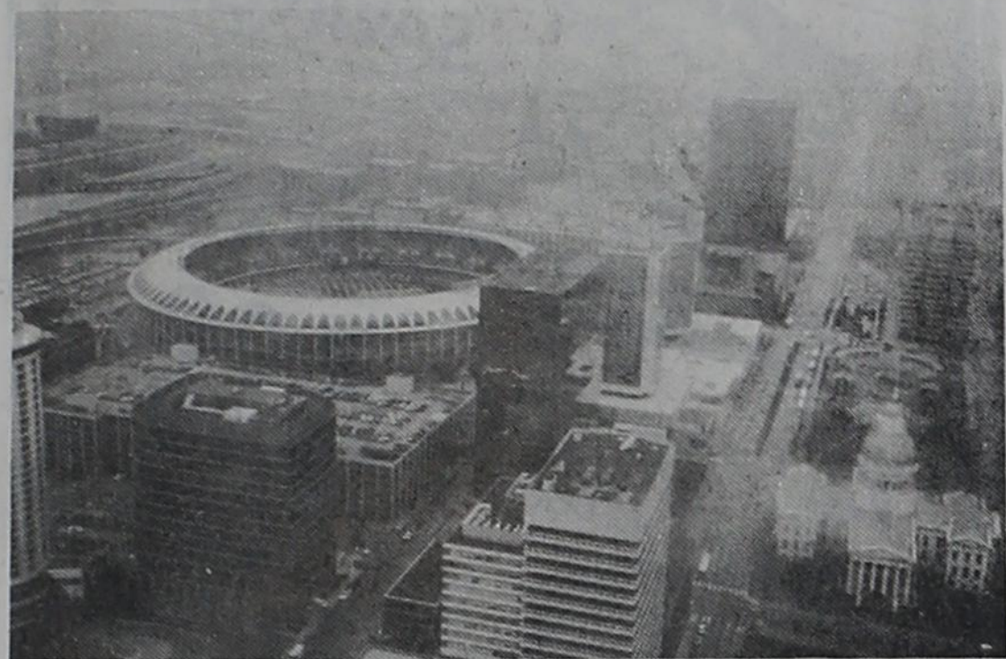
St. Louis skyline as seen from the Arch.
