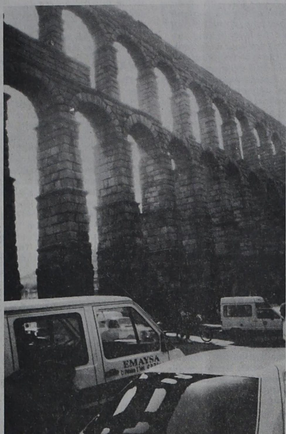
The Roman Aquaduct was built about 1,200 years ago, and is used to convey water from one side of the city to the other. It is built entirely of stone and no mortar of any kind was used in its building. It is still in use today.
