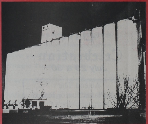
Sherley - Anderson Lazbuddie Elevator
