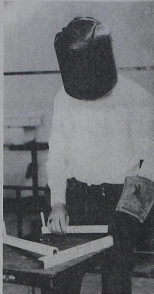
Horner shows how he welded the pieces together.
