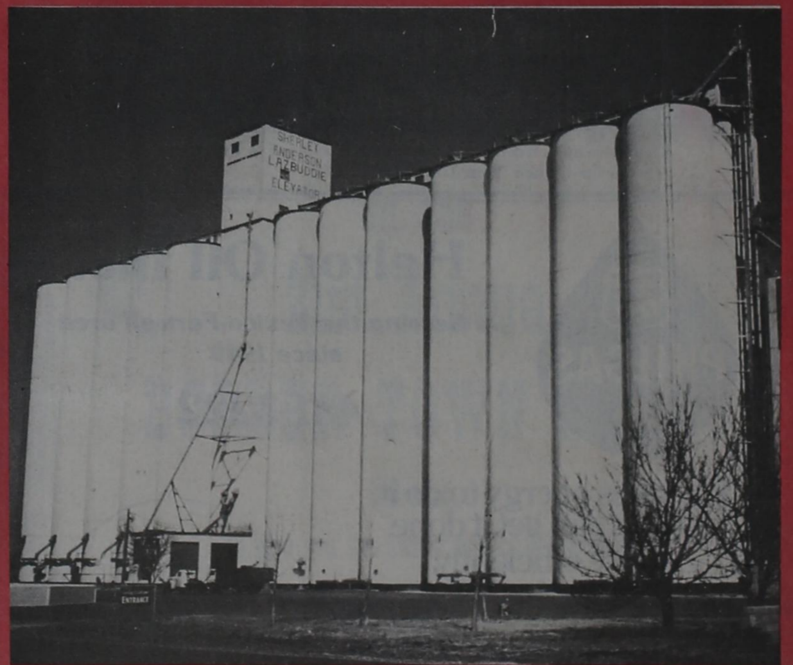
Sherley - Anderson Lazbuddie Elevator
