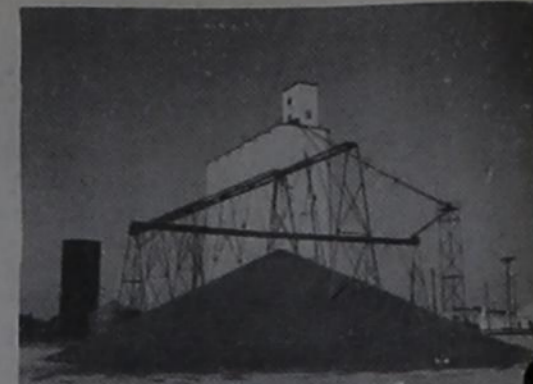
Shown is the grain being put on the ground at the Sherley-Anderson-Pitman Elevator in Farwell.
