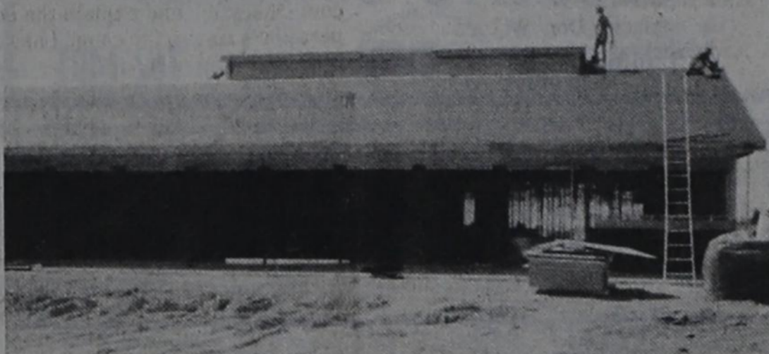
The Town and Country under construction in Texico.
