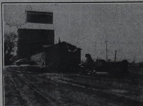
Starting to excavate in Farwell in 1952.
