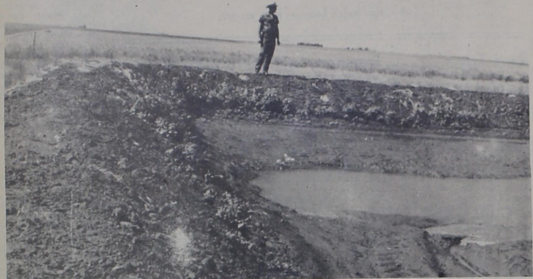
AN EXCELLENT means of curbing tailwater waste is the "low profile" tank, such as the one shown, which is located on the A. L. Hartzog farm south of Bovina. The tank is low
