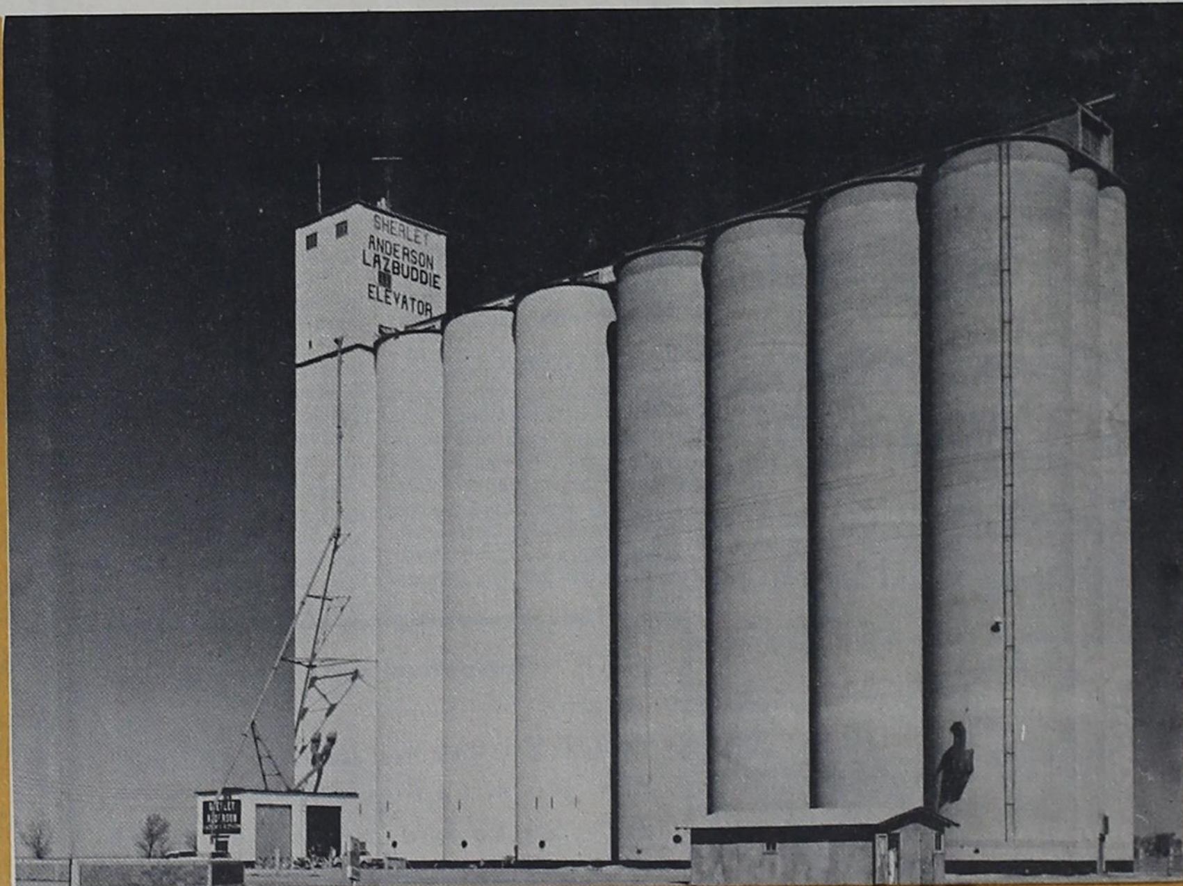
Sherley - Anderson LAZBUDDIE ELEVATOR
