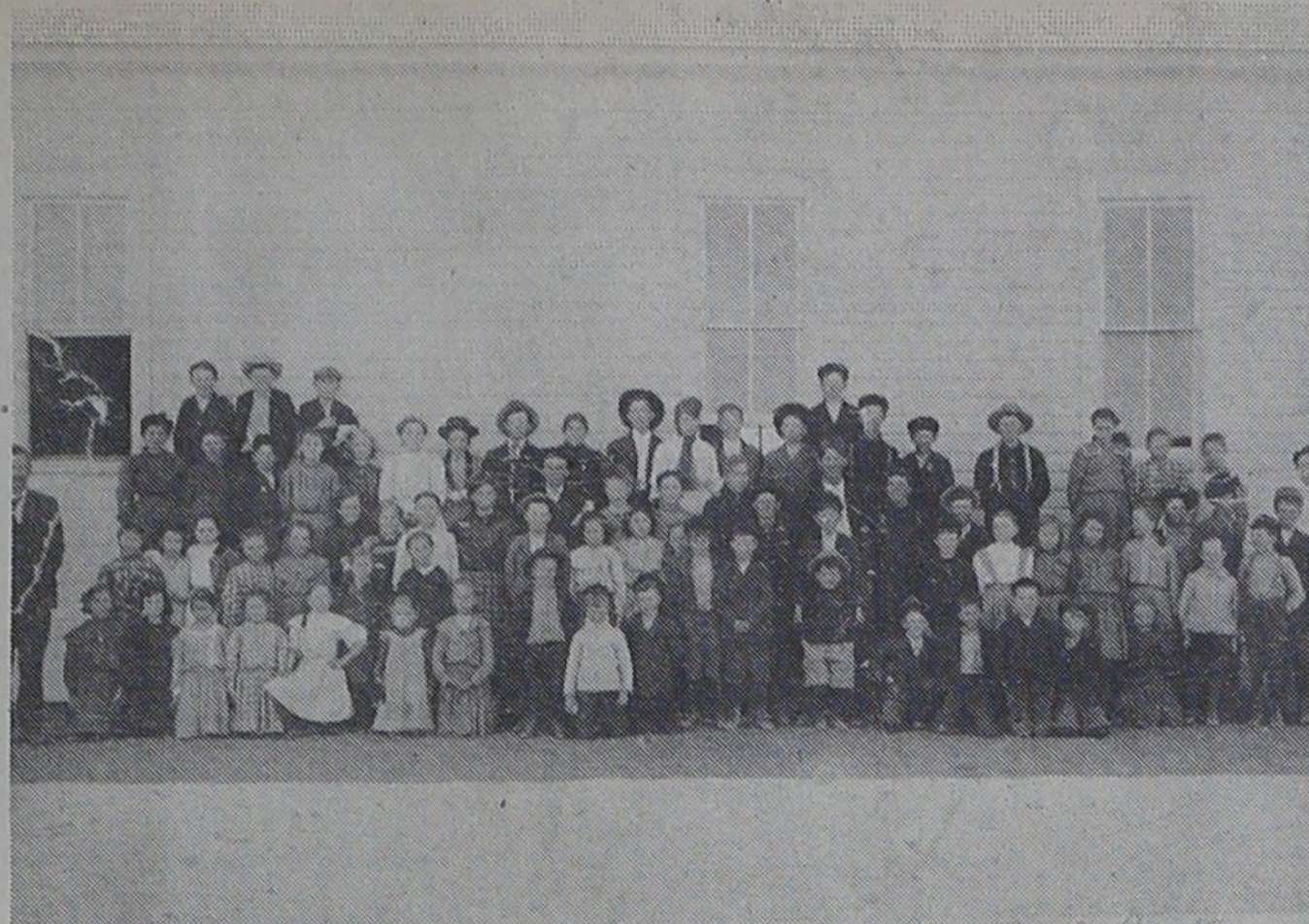
FROM THIS, A ONE STORY FRAME BUILDING CONSTRUCTED IN 1906 . . .
