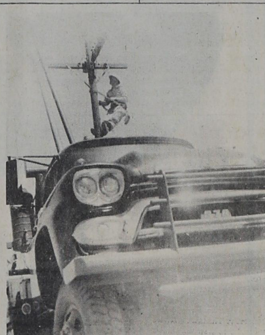
MAKING WAY FOR PROGRESS, these Southwestern Public Service Company workmen were busy moving poles and lines the first of the week in eastern Farwell. They are clearing the way for the paving of 9th Street, which will probably be dubbed "The Loop" by local residents.
