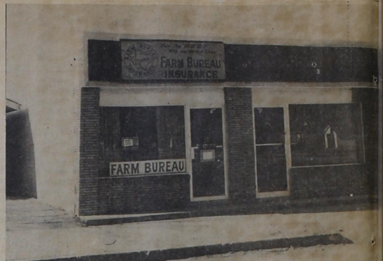
NEW HOME of the Parmer County Farm Bureau is this attractive office building in Friona. It was occupied by the organization and Service Agent Raymond Euler two weeks ago. Garrett, Farwell, is contractor.
