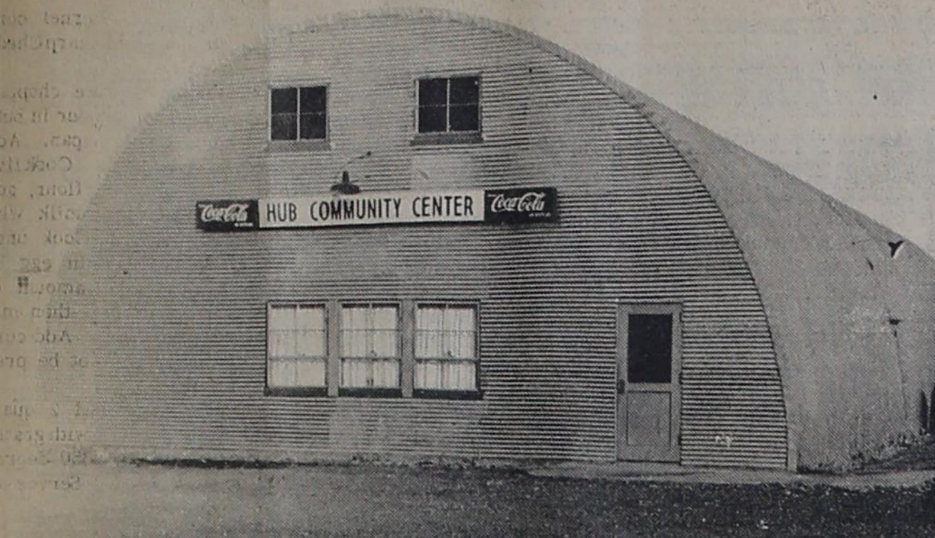
RIGHTLY PROUD are the residents of the Hub Community of this all-steel community center, shown above. It was built two years ago and is the frequent meeting place of farm, civic, study, and neighborhood groups.
