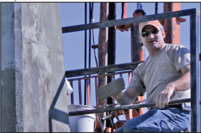
Keith Meeks smooths out the facade.
