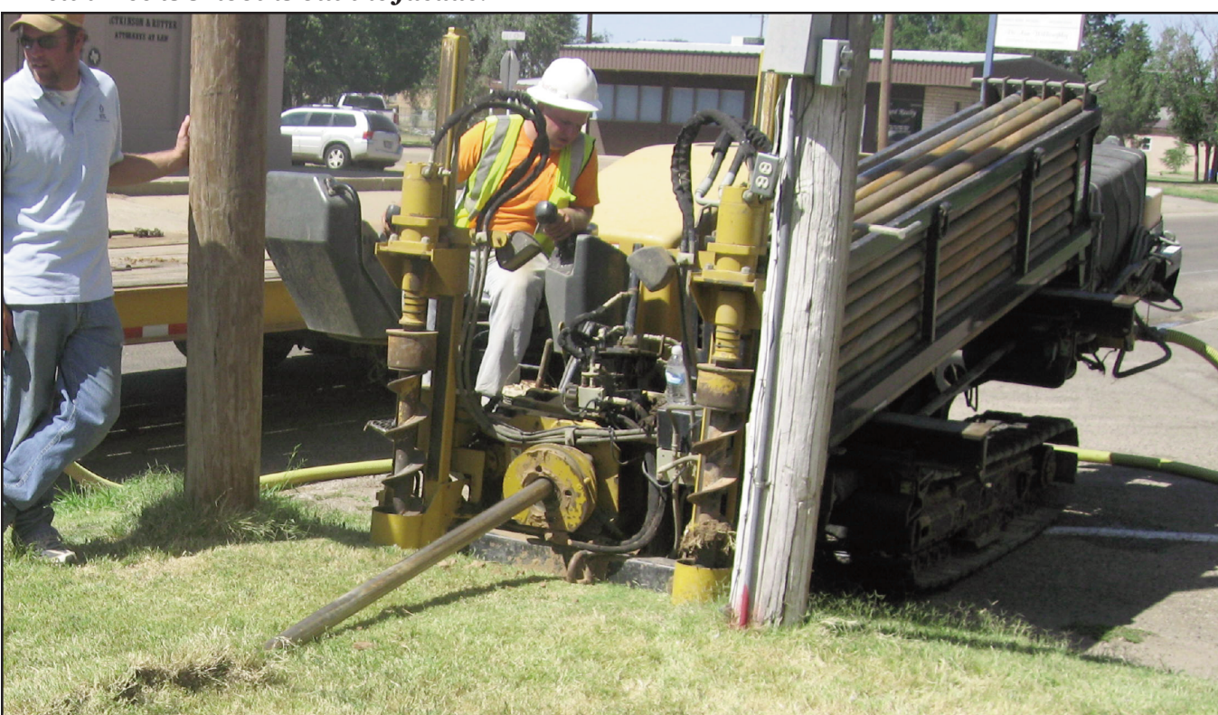
Electricom offered to drill a line to run electricity to the obelisk without needing a trench across the park. The original plan was to build without lights, but this moved up the plans.
