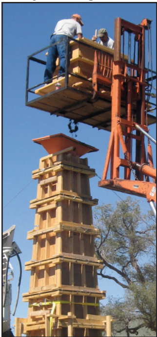
Concrete was poured into this box, then raised to go in the top.
