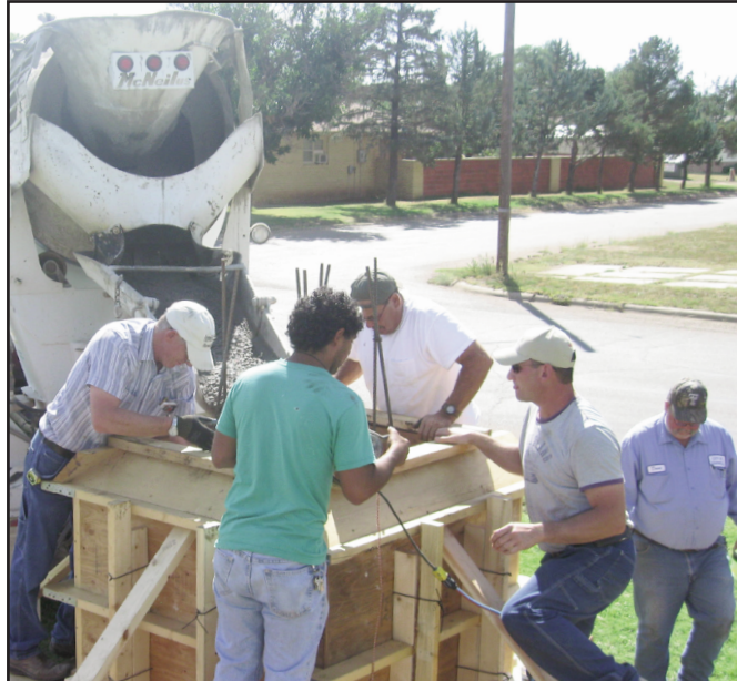
Pouring the first of the concrete.
