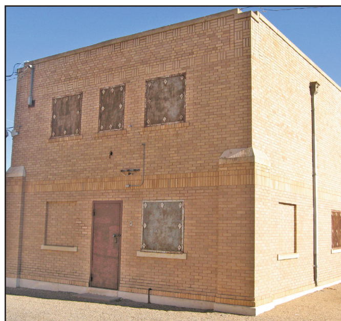
The old Parmer County jail house today is used for the courthouse's storage needs.
