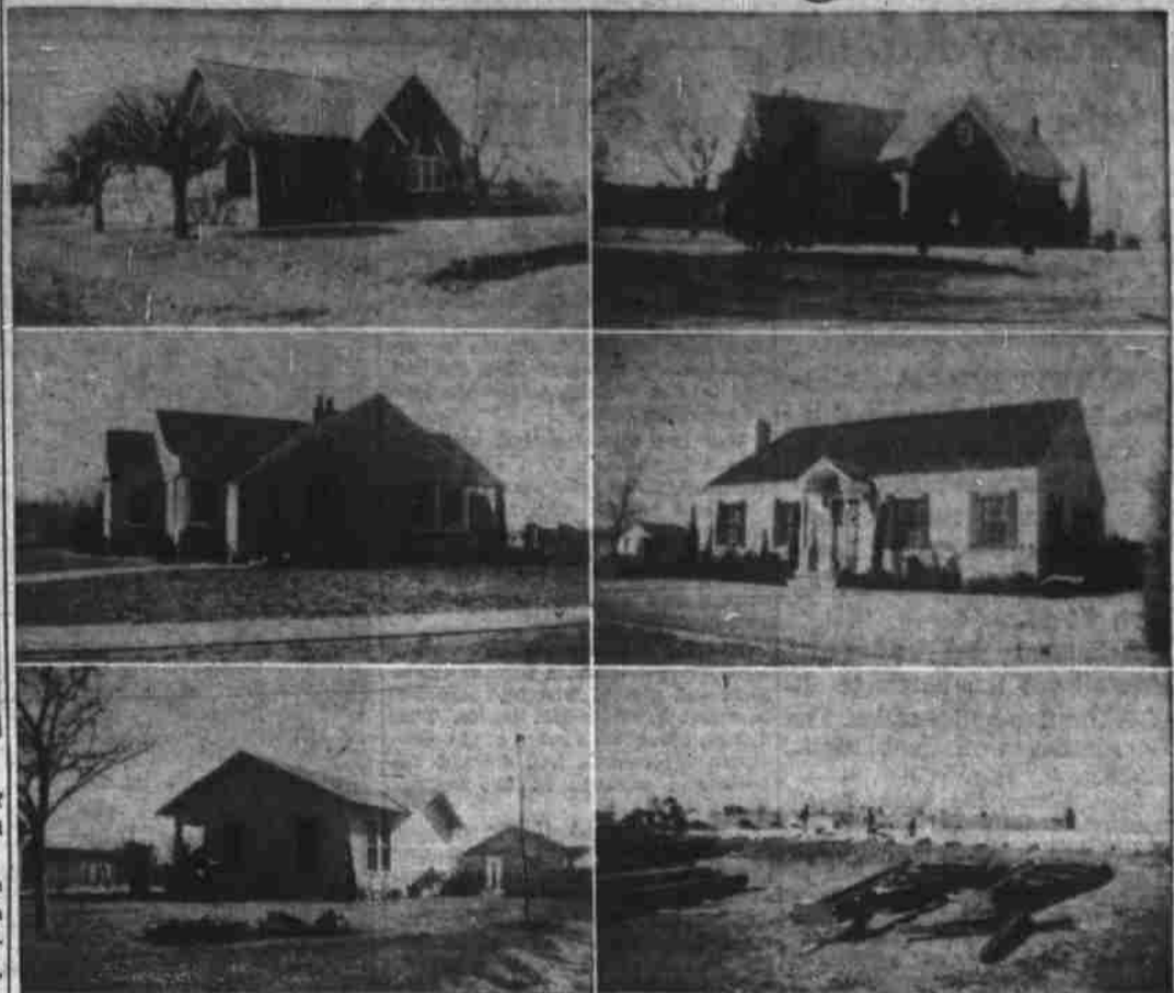
STANTON CONSTRUCTION of the past few years is represented in the above photos. Top left, the home of Mr. and Mrs. Y. Y. Houston, and right, that of Mr. and Mrs. Sam Turner. In the middle panel, the Ernest Price and Poe Woodard residences. Left below is the home of Mr. and Mrs. Wayne Moffett, and at the right a scene of the start of construction on Stanton high school's new gymnasium.
