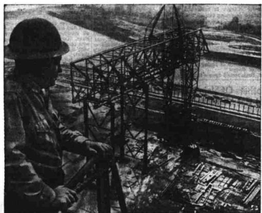
NEW STEEL MILL TAKES SHAPE — Construction worker on lofty perch views part of U. S. Steel Corporation's new Fairless Works along Delaware River near Morrisville, Pa. In center is framework of bridge designed to carry ore from boats docking along river bank. The \$450,000,000 plant, started little more than 19 months ago, expects to produce first steel in December.
