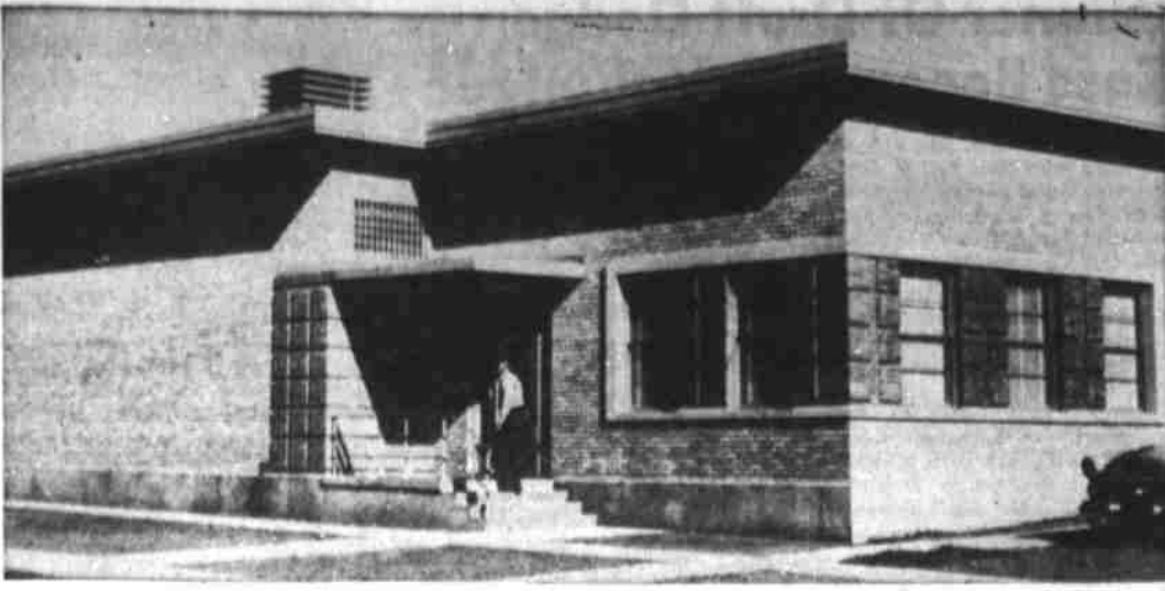
NEW TELEPHONE BUILDING TO GO ON DISPLAY An early visitor is Bob Hamrick, Colorado City postman
